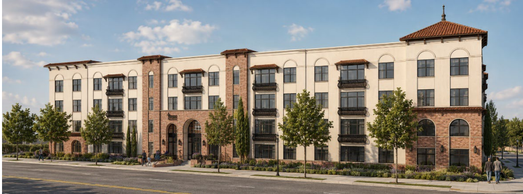
Exterior view from S. Monaco Parkway
